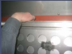
Chamber roof removed showing damper
