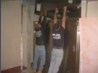
6. Lowering upper section onto assembled chamber
