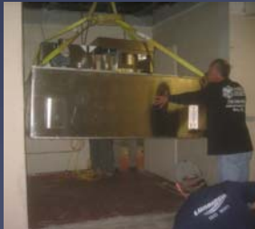
3. Hoisting upper assembly
