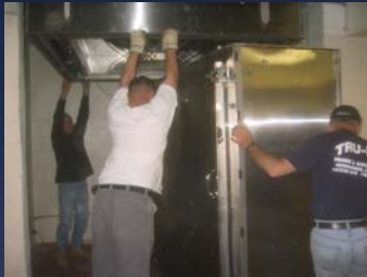
5. Positioning chamber in wall opening
