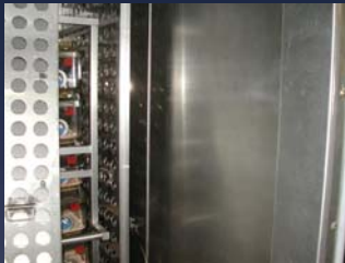
One sidewall panel removed
